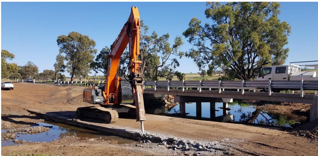
Billy Kings Creek Bridge Project
